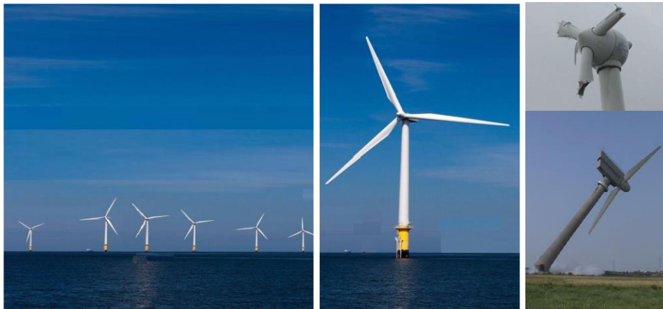
Fig. 1(a) quest for design and construction of giant offshore wind turbine: Giant single wind turbine as opposed to wind turbine farms; (b) broken wind turbine blades and stability problem (C.C.K., Belgique Tournai - Bruges - région de Courtrai)
